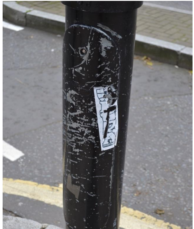
Tavistock Place. Partially removed sticker with damage from metal scraping.
